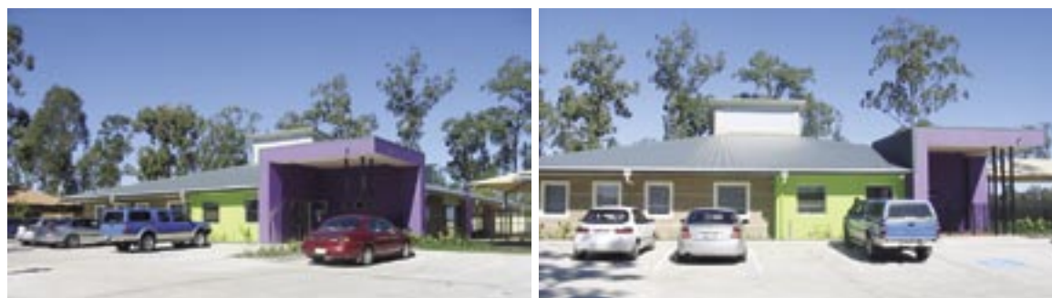
Figure 5 – Typical Existing Centre Purchase
